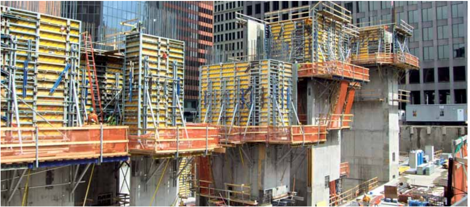
The modular and symmetrical panels of the Framax Xlife ensure the best possible utilization of formwork.
