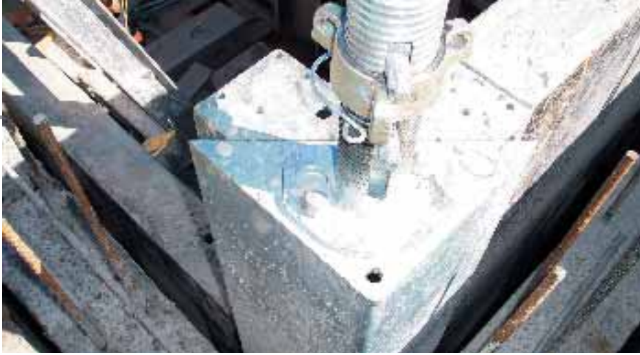
The new Framax stripping corner I makes for particularly efficient forming of shafts.
