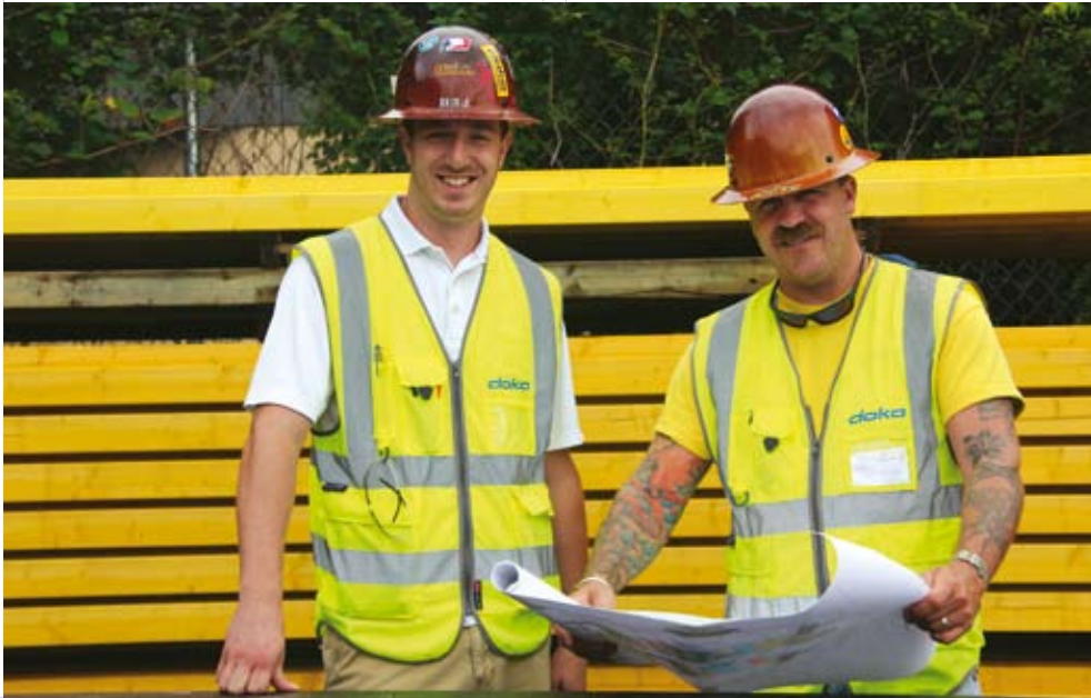
▲ Ron Moyer and Rich Barton support crews at Ground Zero in handling formwork to maximize safety and increase efficiency.
