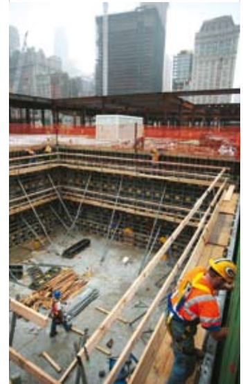
▲ Doka provided detailed engineering drawings to ensure the best possible utilization of formwork was achieved. ▼
