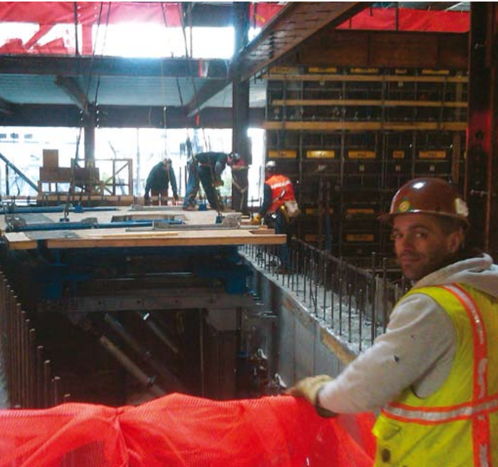
▲ To climb the inside of the tower's main core, a combination of automatic climbing formwork SKE 100 and Xclimb 60 is being used. Additionally, SKE 100 is in use on the perimeter of the building to climb the concrete mega-columns. The SKE 100 system, which can carry 27,000-pounds per bracket, was ideal for handling the bigger loading platforms that were required for certain areas. Doka's Xclimb 60 uses lightweight hydraulic units, quickly lifting up to four brackets simultaneously.
