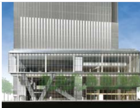
▲ Frami framed formwork was used to create the architectural “V-columns” on Tower 4 due to its lightweight flexible, hand-setting capabilities.
