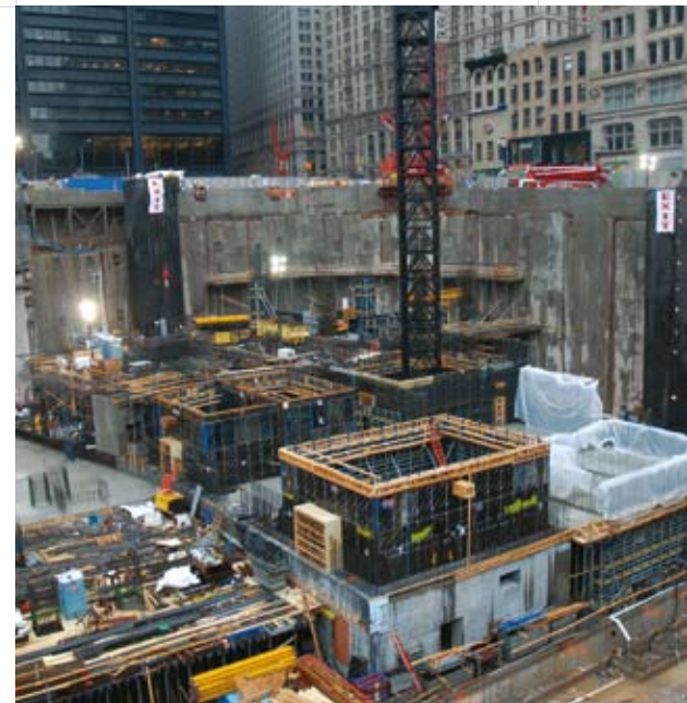
▲ The Tower 4 footprint area of the elevator cores was broken down into four quadrants in order to achieve the best productivity from the labor force.
