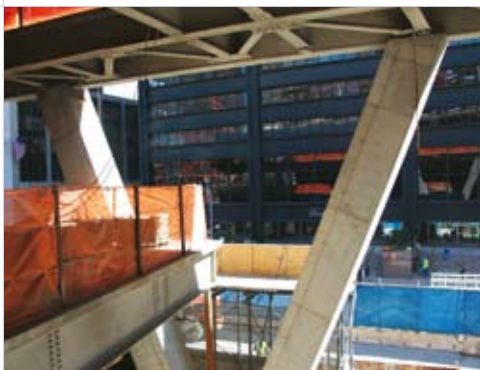
▲ Frami framed formwork was used to create the architectural “V-columns” on Tower 4 due to its lightweight flexible, hand-setting capabilities.
