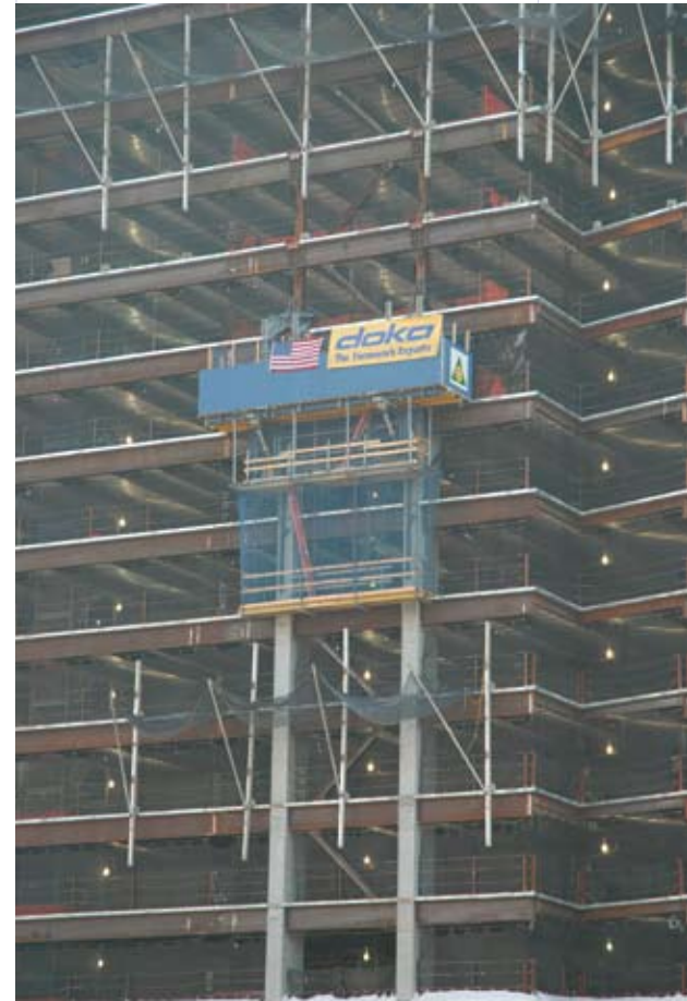
▲ To climb the inside of the tower's main core, a combination of automatic climbing formwork SKE 100 and Xclimb 60 is being used. Additionally, SKE 100 is in use on the perimeter of the building to climb the concrete mega-columns. The SKE 100 system, which can carry 27,000-pounds per bracket, was ideal for handling the bigger loading platforms that were required for certain areas. Doka's Xclimb 60 uses lightweight hydraulic units, quickly lifting up to four brackets simultaneously.
