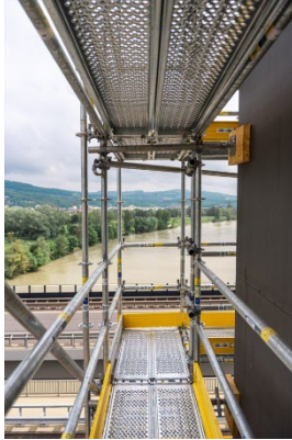
Ringlock scaffolding system in use for the renovation of the cable-stayed bridge on the River Danube. Copyright: Clean Frame Photography
