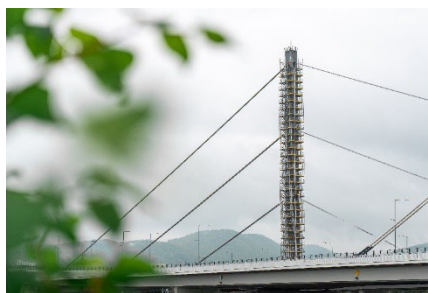
Ringlock was used to scaffold the 65-metre-high pylon of the Voest Bridge in Austria.
