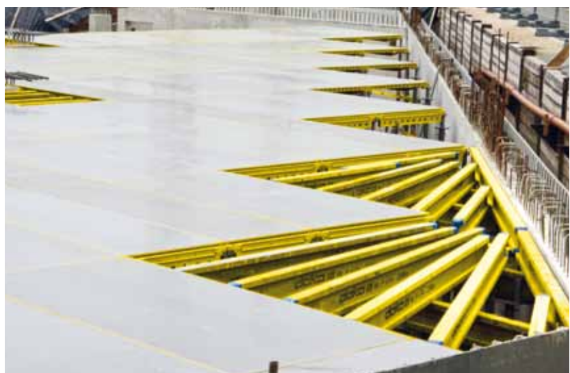
▲ With the suspension clamp, infill zones can be formed quickly and easily, as Dokadek 30 merges here seamlessly with Dokaflex.
