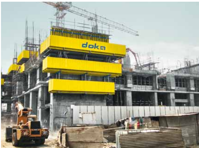
▲ Automatic climbing formwork SKE50/100 for working at elevated heights.
