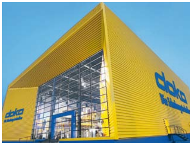
Doka showcased some pathbreaking formwork-technology innovations at bauma 2010 in Munich.
