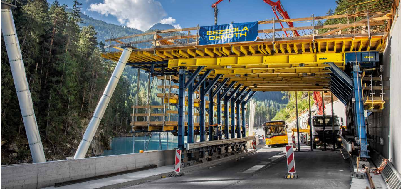
Mingør Gallery | Switzerland | Doka UniKit primary beams and extensions
