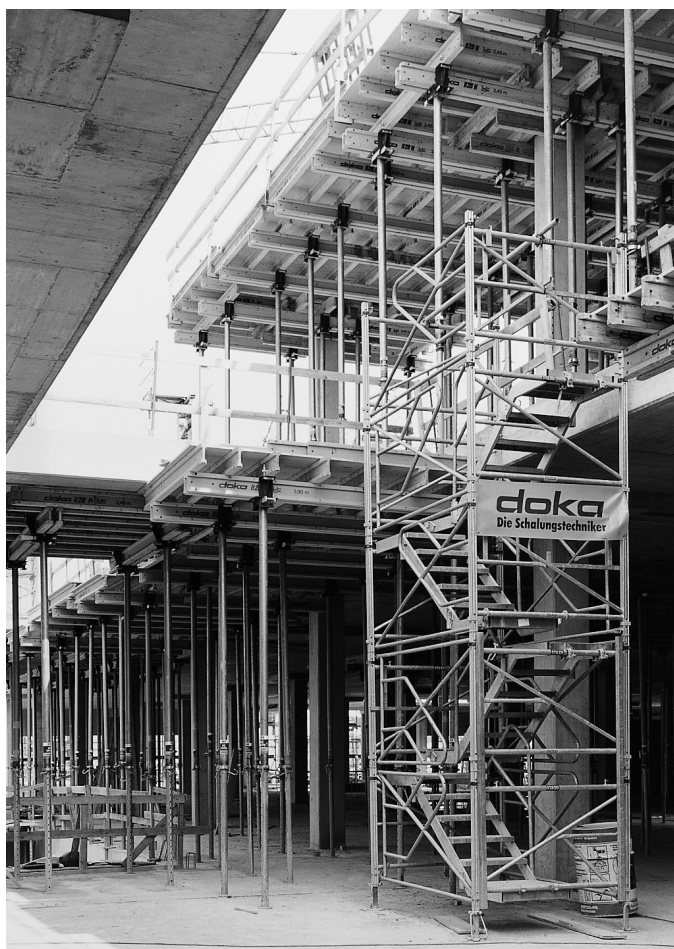
Obra: ARGE Westmünster Center, Bocholt
