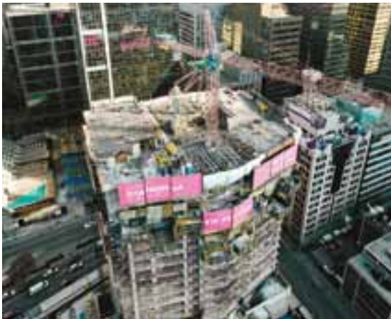
Doka's Protection Screen provides premier protection for the working floor and the three floors below at the site of Shangri-La Hotel, Toronto, ON
