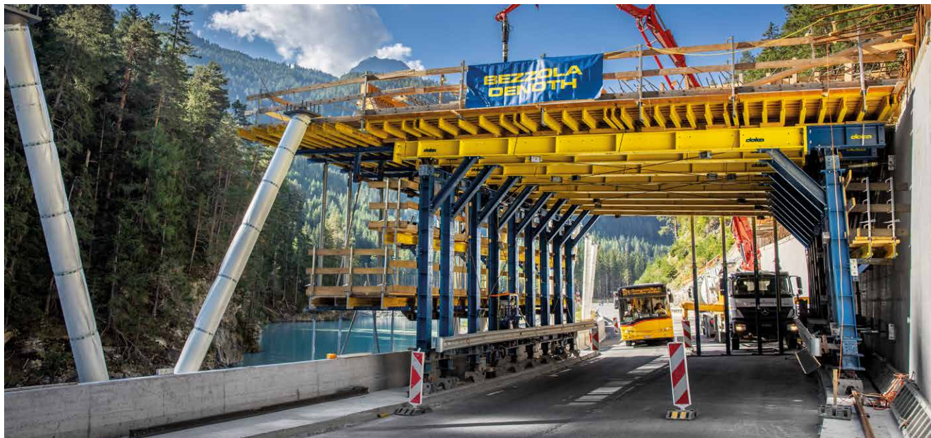
Mingèr Gallery | Switzerland | Doka UniKit primary beams and extensions
