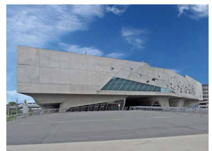
Fair-faced concrete projects
