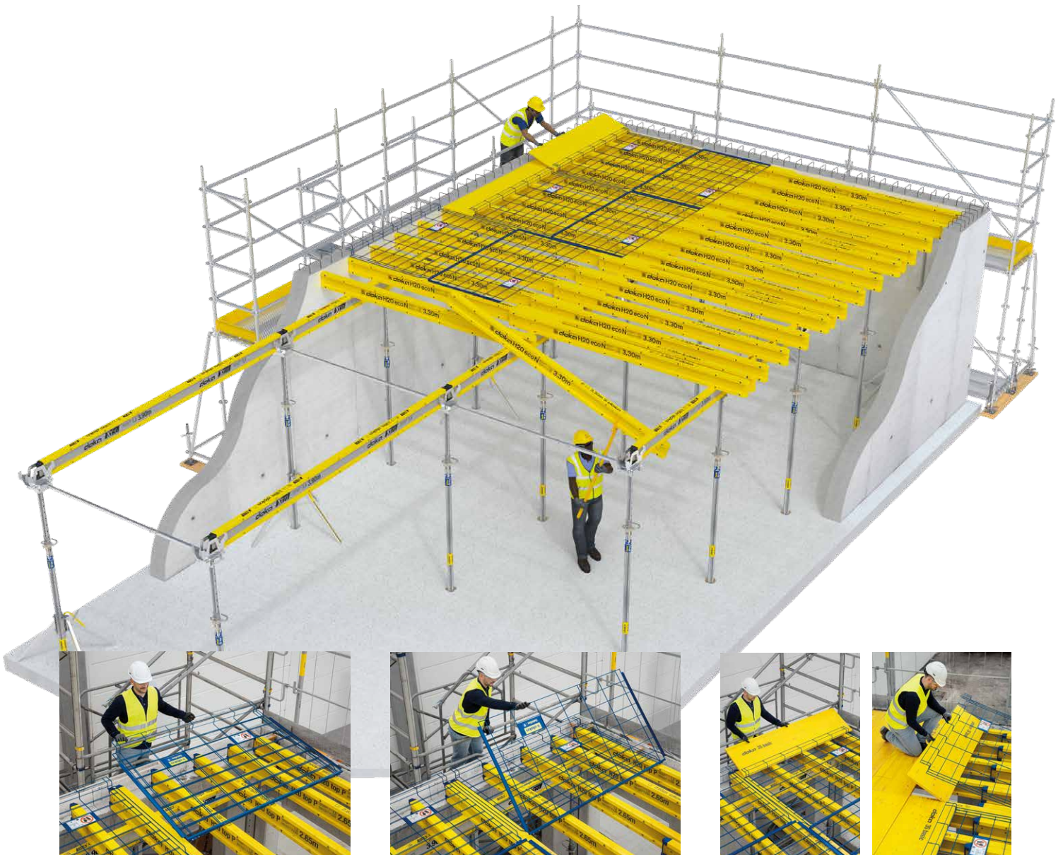
1 Lay mesh in position
