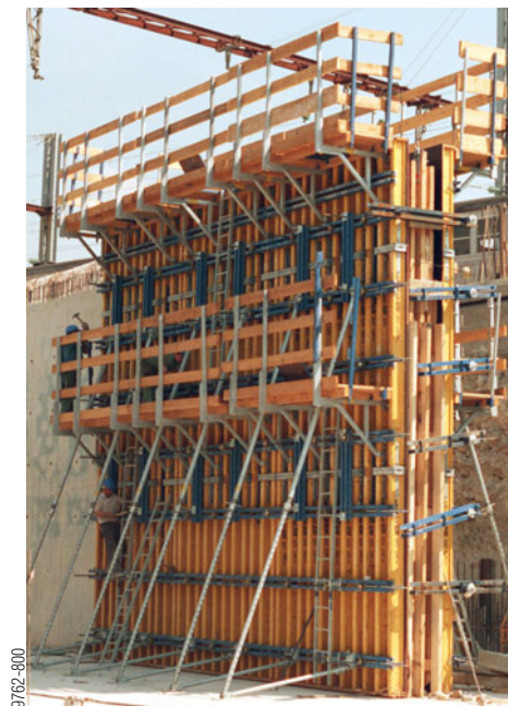
Baustelle: TVG Nord Bridge No. 4, Paris
