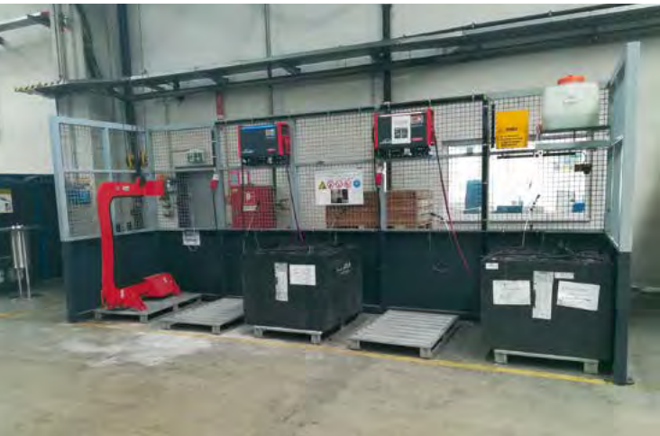
Charging station for exchangeable batteries
