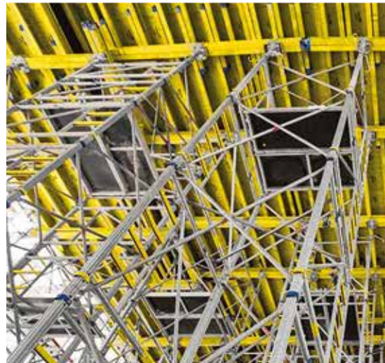
Lightweight scaffold planking units made of aluminium, and a built-in anti-liftout feature, make for safe assembly and safe working conditions inside the scaffold.
