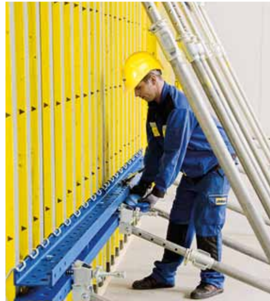
Having only a few different connecting and anchoring components speeds up the workflow.
