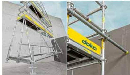
The widened support base of the bracing scaffolding, and the fact that it is braced against the formwork, give it greater safety against tipover.
