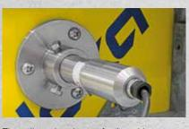
The wall sensing element for the cable sensor is incorporated directly into the form-facing and repositioned together with the formwork.
