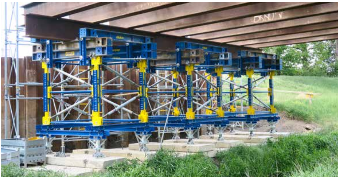
UniKit shoring towers with load-bearing capacity of up to 480 kN per leg.
