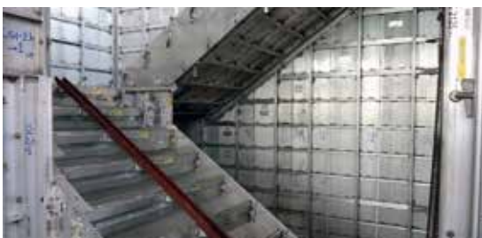
▲ Thanks to test assembly we can every time ensure the correct setup of the system - especially for special areas like as staircases, special shaped walls, etc.
