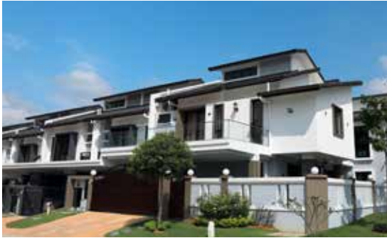
▲ 150 Mid-range linked townhouses in the Shah Alam area in Kuala Lumpur
