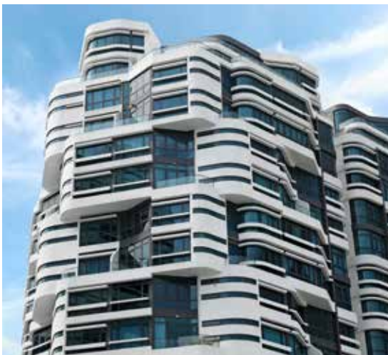
▲ Multi generational and harmonious residential sanctuary, where a cycle time target of 5 days per floor was achieved due to the formwork solution.
