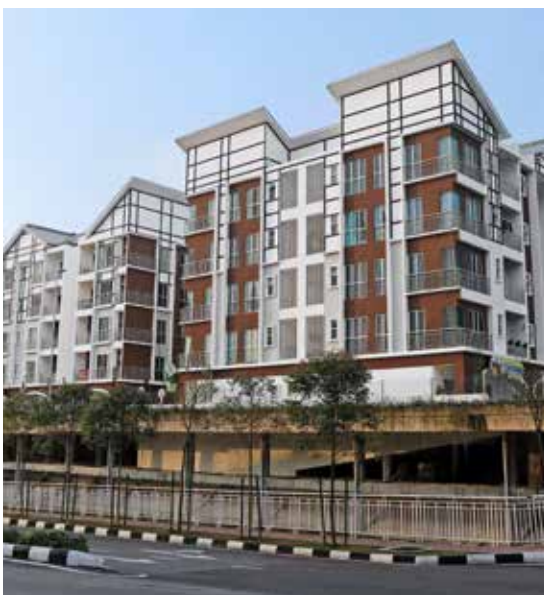
▲ Cameron Highlands, Summer Square comprising ground floor and 4 storey low rise apartment buildings with retail at ground level. Retail units cast first and apartment floors completed at a rate of one floor every 5 days.
