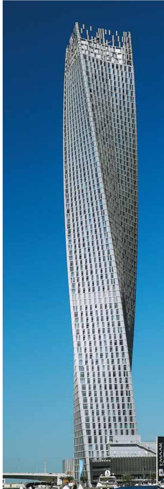
▲ The Cayan Tower, a luxury apartment building with a striking helical shape, turning 90 degrees over the course of its height.
