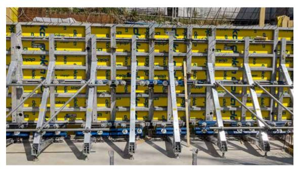
$\textbf{Compatibility with Dokas framed formwork systems allows to use the Supporting Construction Frame AL\ all\ areas\ of\ application.}$
