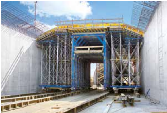
▲ Load-bearing tower Staxo 100 combined with Tunnel formwork system SL-1
