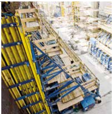
▲ Supporting construction frame mounted on travelling unit
