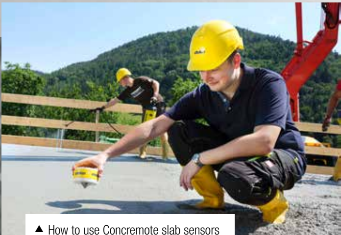
▲ How to use Concremote slab sensors
