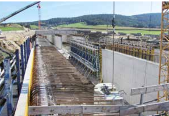
▲ Large-area formwork Top 50
