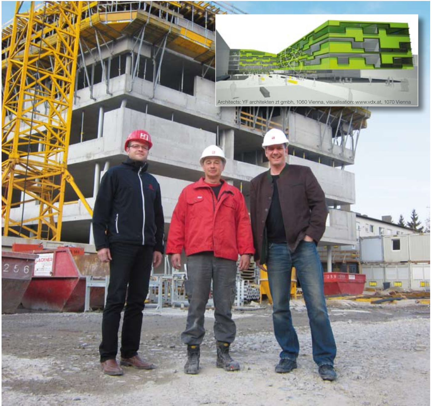
The Aigelsreiter team, left to right: Construction engineer Christian Absenger, lead foreman Anton Hudl, managing director Ernst Aigelsreiter.
