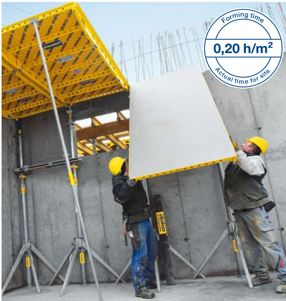
The rectangular panels make even high-level slabs easy to form.
