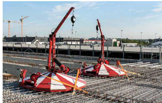
FreeFalcon PCC has been specially developed for use on sectional slabs and secures workers on the slab edge while assembling the sectional slabs.
