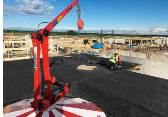
The FreeFalcon protects construction crew members whenever work at drop-off edges is temporarily unavoidable.
