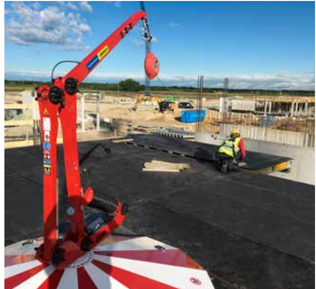
The FreeFalcon protects construction crew members whenever work at drop-off edges is temporarily unavoidable.
