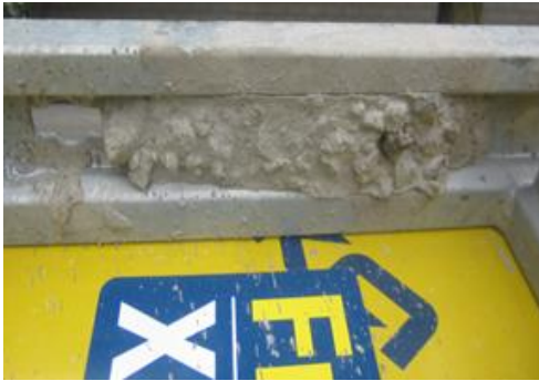
Inner frame profile filled with concrete
