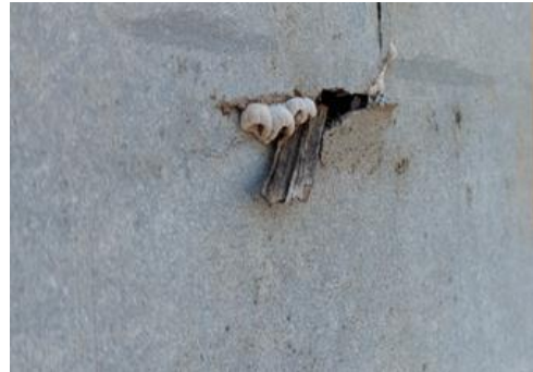
Holes + drills diameter > 2 cm
