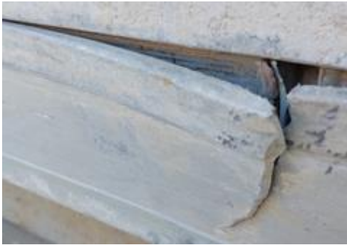
Length profile broken
