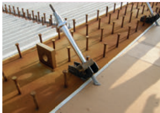
The 'ParaTop insert-shoe - steel' with the re-useable ParaTop insert-cone
