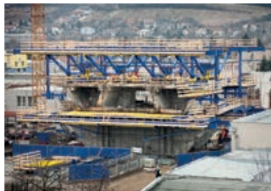
Nitra Bridge, Slovakia
