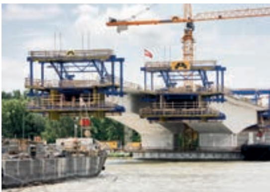
Danube bridge at Traismauer, Austria
