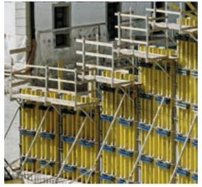
The practical height grid and the systematic spacing of the form-ties make it possible to form widely differing height-combinations quickly and easily.
