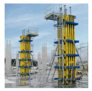
Used in conjunction with the Doka column formwork platform 150/90cm, the Ladder system XS ensures high worksite safety.
