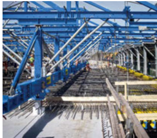
The new System beam NG allows the Composite forming carriage to be adapted to the structure geometry even more flexibly.
