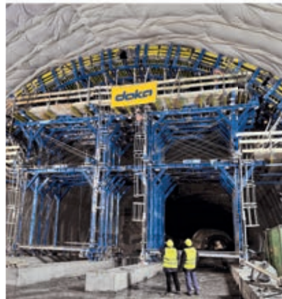
The Heavy-duty supporting system SL-1 is also easy to adjust to very wide tunnel arches.
