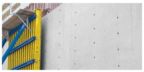
Key architectural specifications can be fulfilled with the Top 50 system, as it allows a free choice of form facing and form-tie pattern.
