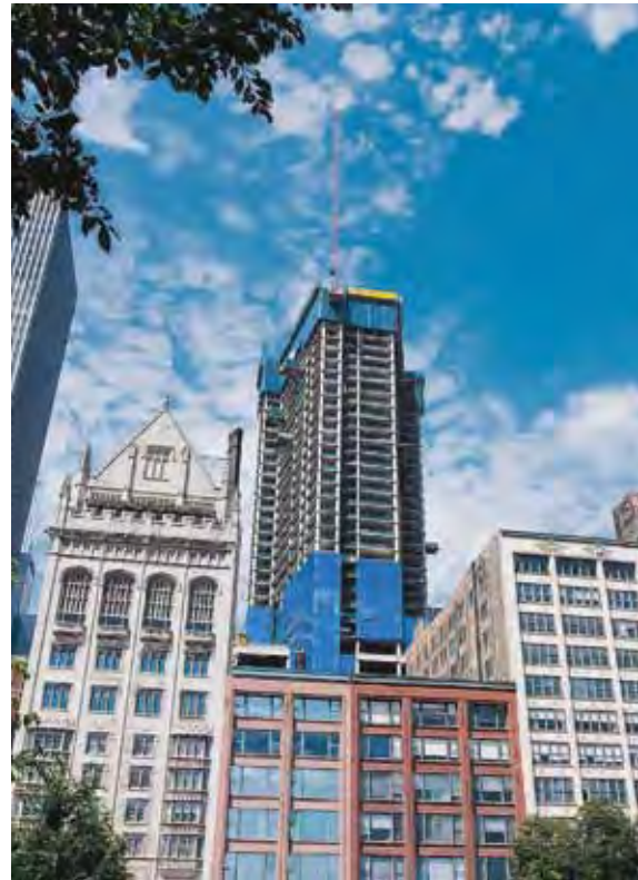
The Protection Screen Xclimb 60 provides full highrise perimeter protection at the Legacy Tower, Chicago.
