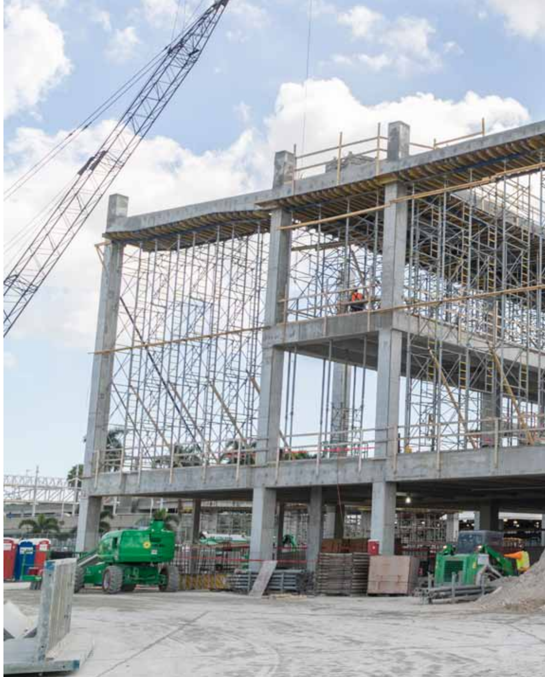
▲ Load-bearing tower Staxo 100 and Dokamatic Tables in use on the 250,000 sq. ft. airport terminal expansion.
