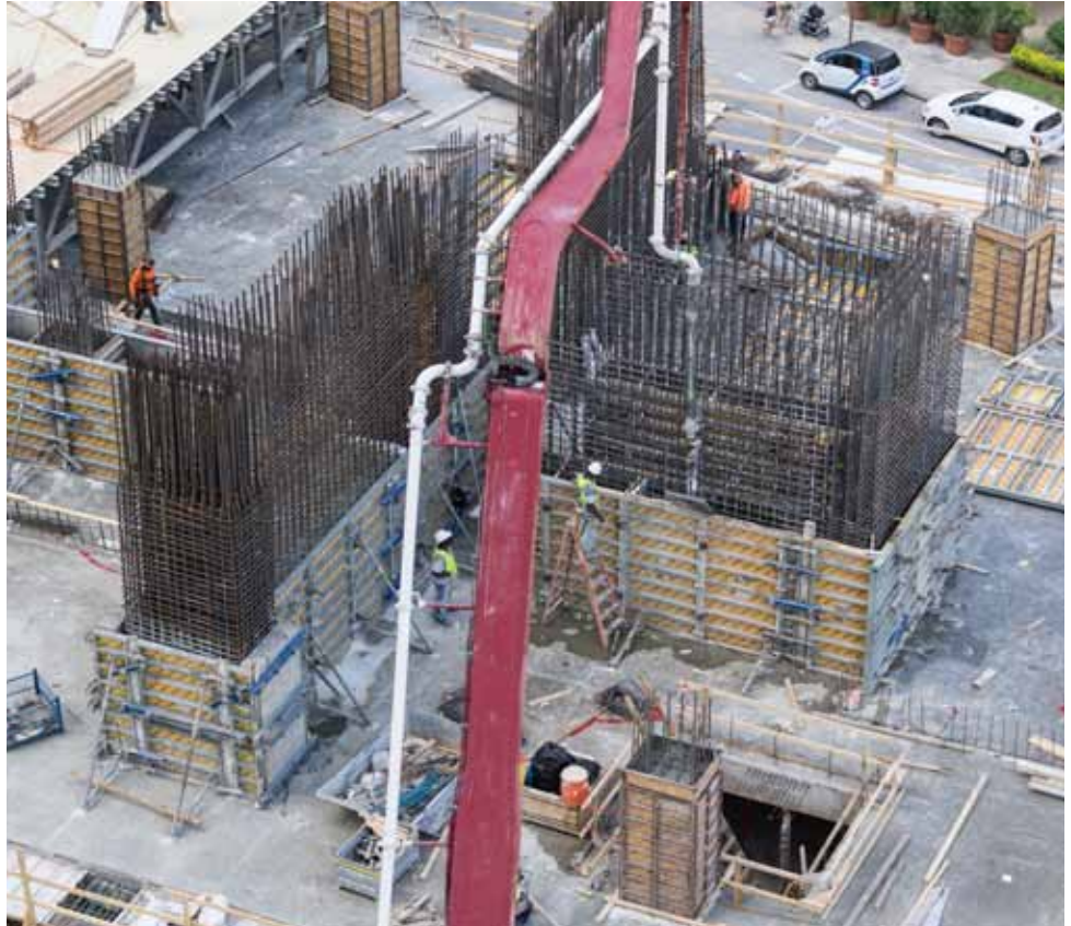
▲ The integrated Framax stripping corners and shaft platforms allowed the contractor to strip and lift the stair and elevator cores in one crane pick.
