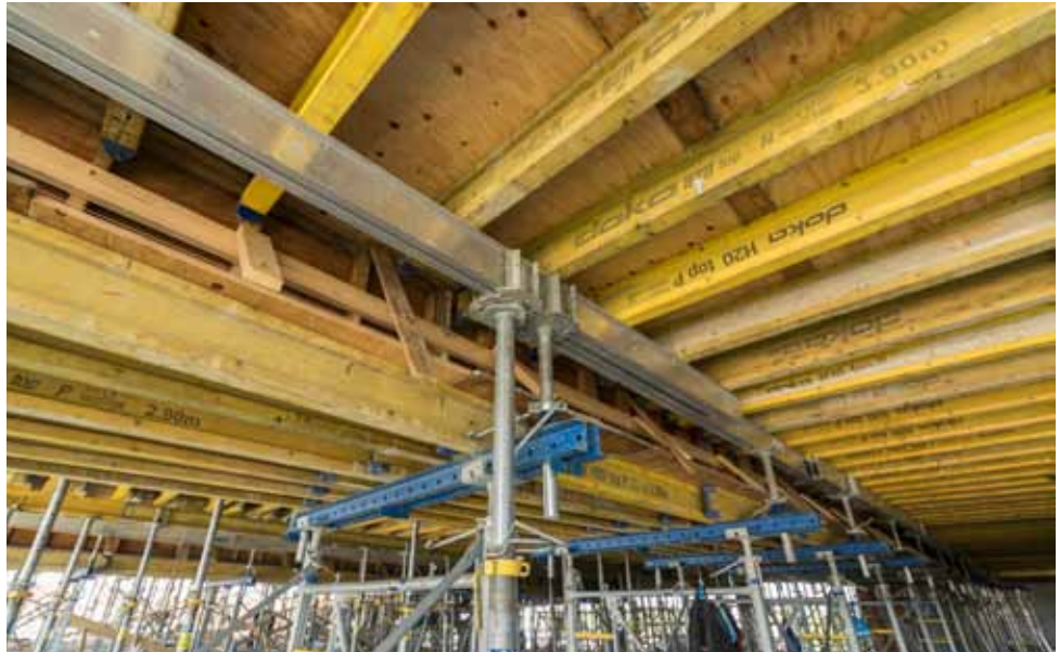
▲ Doka fabricated custom mounting brackets. This allowed Teitelbaum to form the beams which permitted the upper deck to be supported by the head below without any additional materials.
