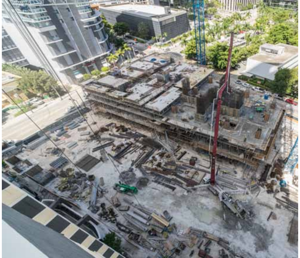
▲ The biggest challenge for the customer was to find a panelized wall formwork system that would be easy for the working crew to learn, use, and reconfigure.
