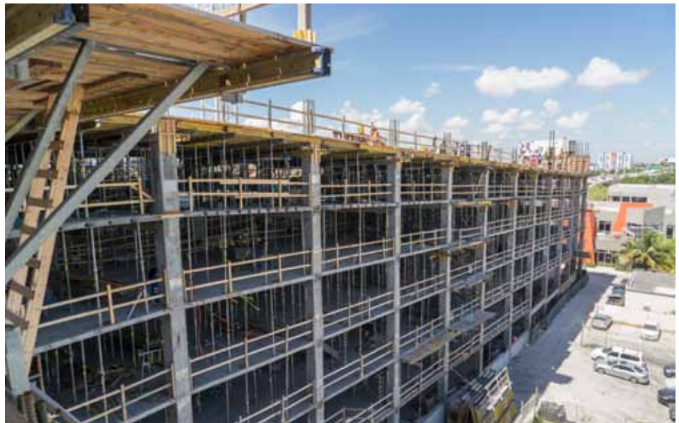
▲ A combination of Dokaflex, MF240 platforms, interior shaft platforms, Platform K and the Top 50 system were used to complete this 5 story parking garage.
