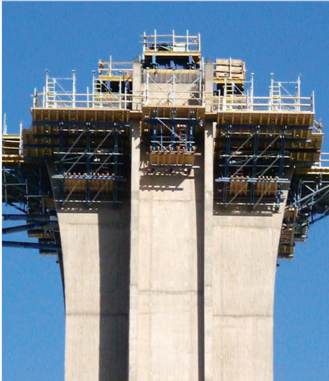
▲ Large area Top 50 formwork together with self-climbing SKE 50 plus, used on the exterior walls, and the Super Climber system, used on the interior walls, provided a fast cycle with a superior architectural concrete finish.
