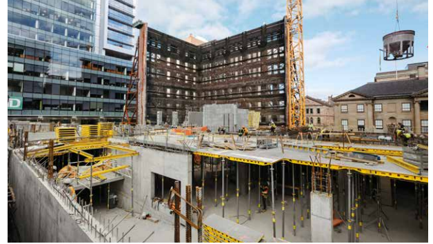
Doka Halifax's Press Block project required the use of our Dokadek 30 and a single sided Framax Xlife plus application to preserve the existing historical facade of the building.
