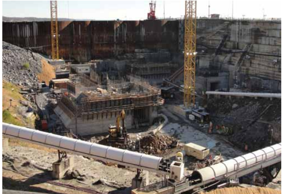
▲ Construction of large mass concrete monoliths takes place for a new upstream lock addition on the Tennessee River.
