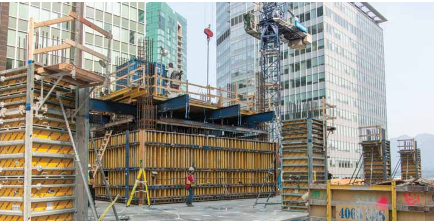
▲ Super Climber SCP in place for its first use in Vancouver, Canada.
