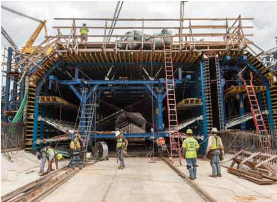
▲ The modular design of the heavy-duty SL-1 components support the heavy loads of each tunnel segment with minimal deflection.
