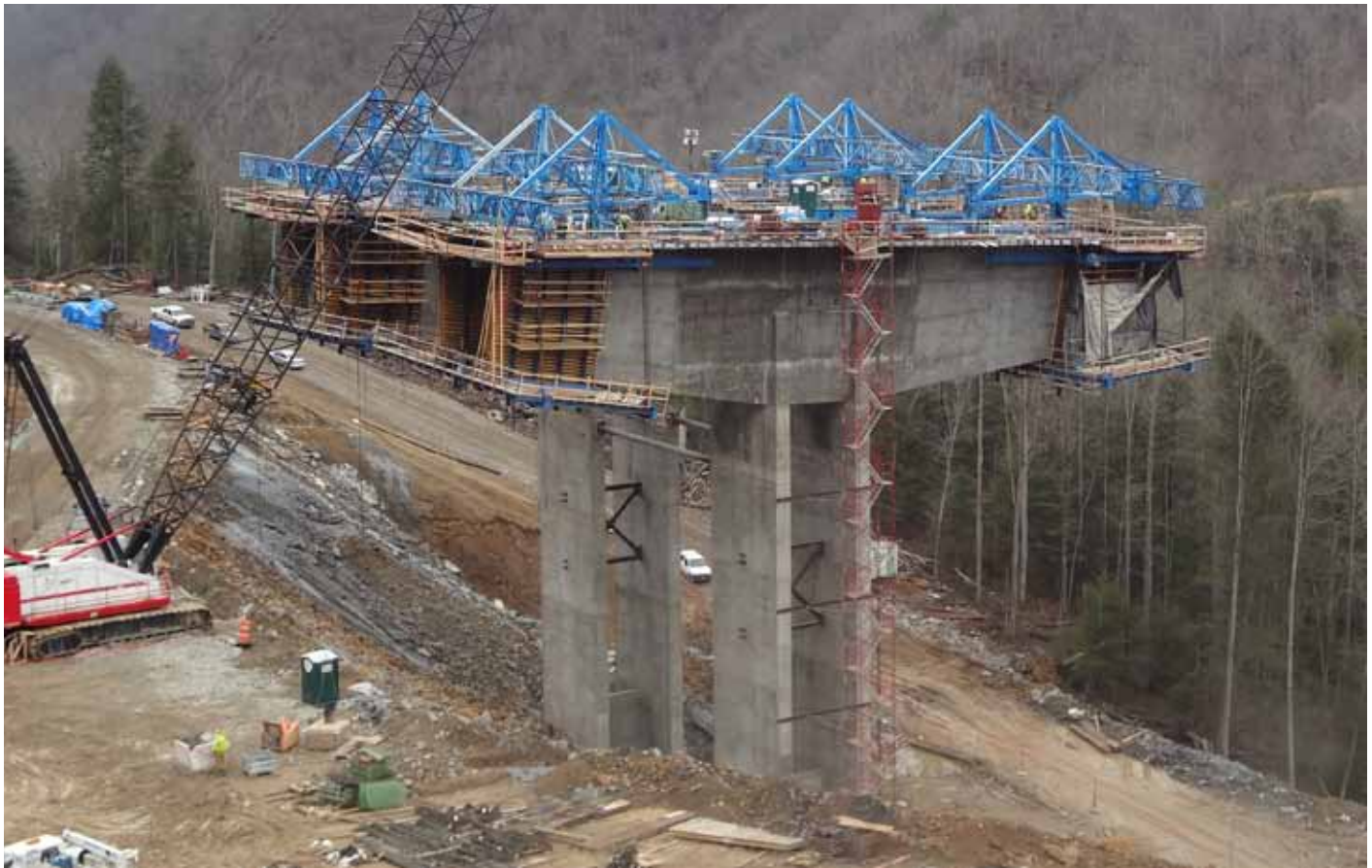
▲ Form travelers by VSL support Doka's versatile Top 50 formwork for variable depth cast-in-place segments.
