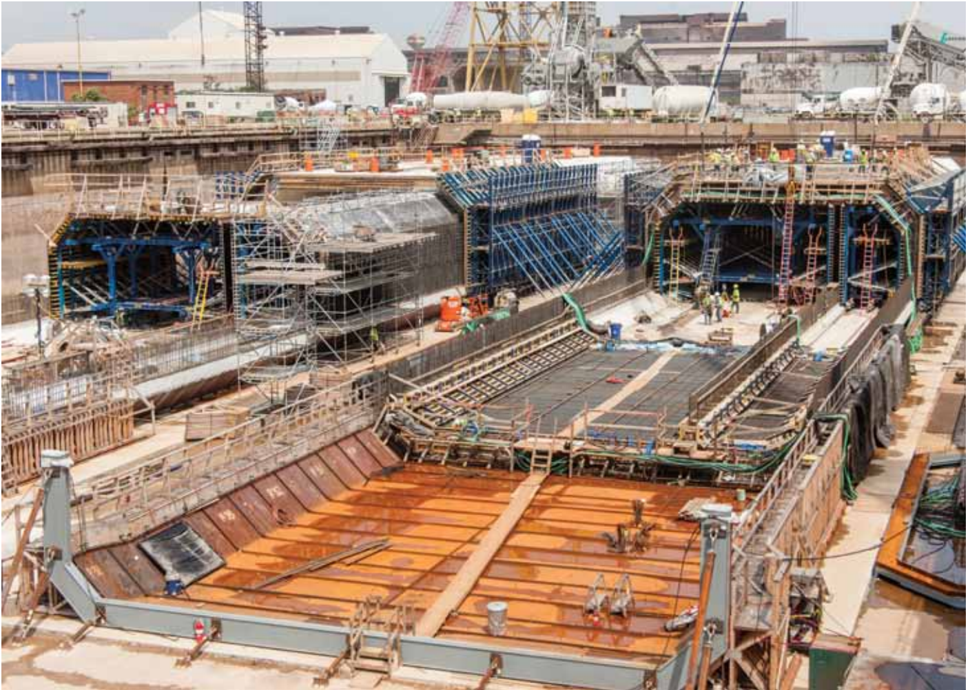
▲ Tunnel segments each weighing nearly 13 tons are precast in a dry dock near Baltimore, Maryland.
