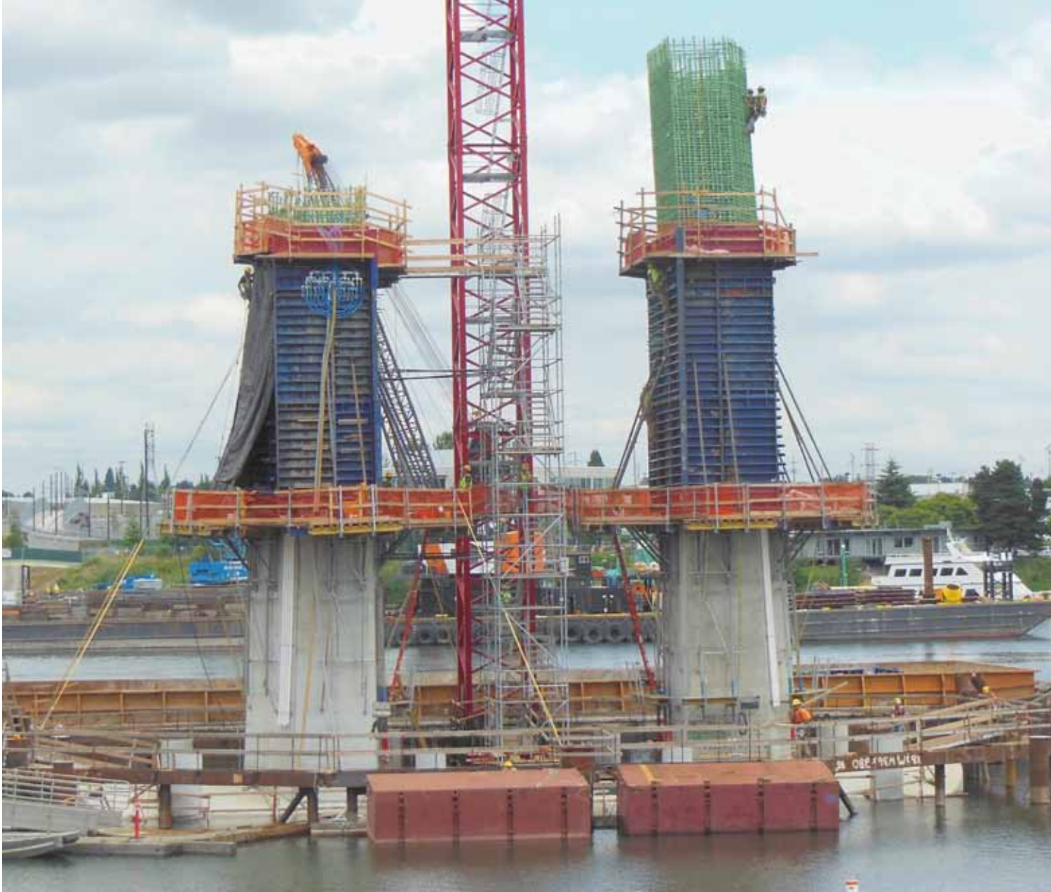
▲ Doka's Steel Girder formwork used in conjunction with MF240 climbing platforms to construct the second 30' tall lift of each pylon.
