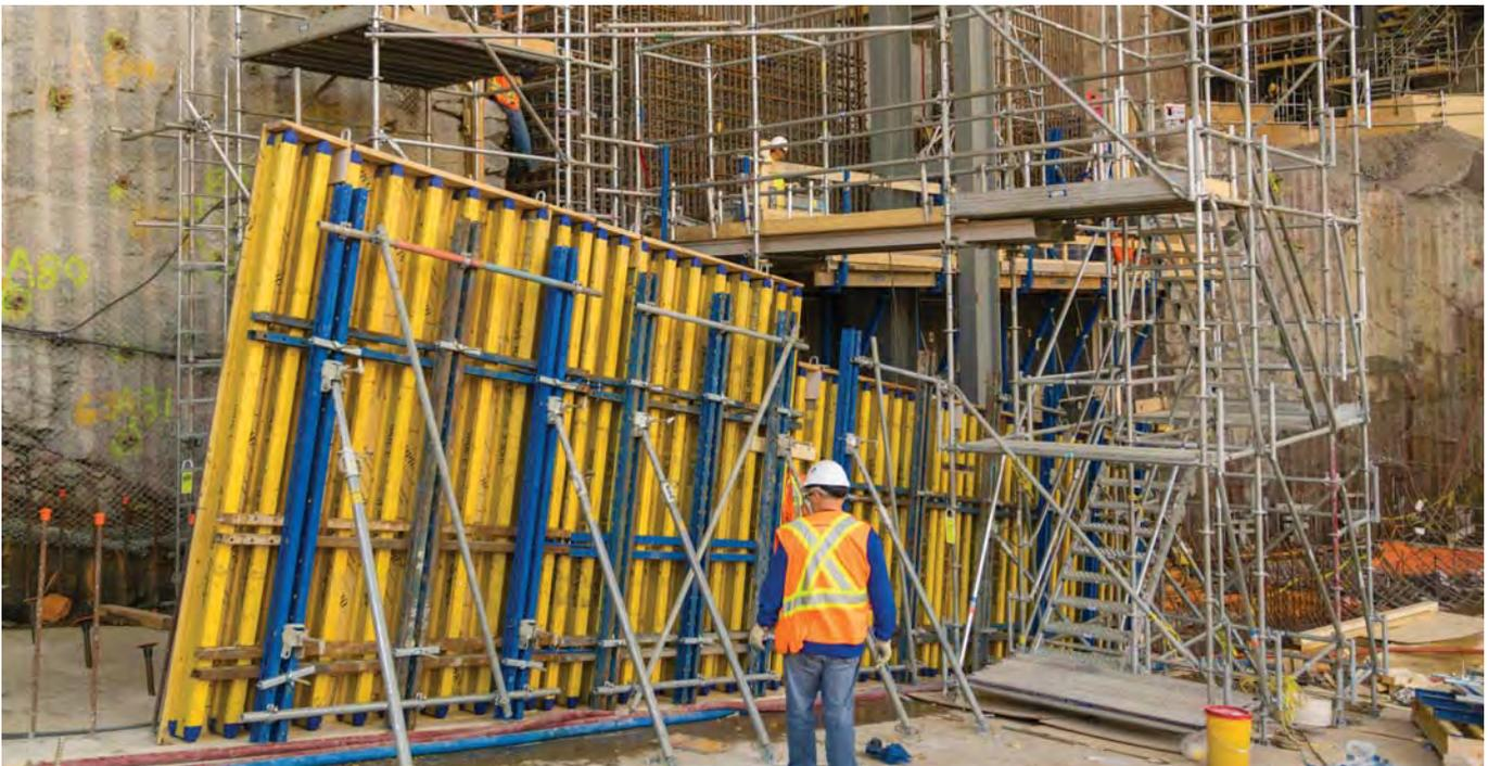
▲ Formwork installed on sloping base slabs and poured against bedrock
