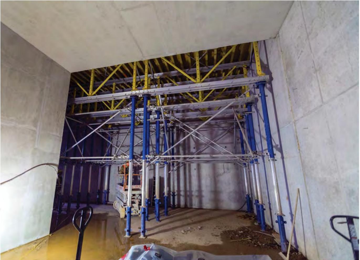
▲ 5.9 m shoring height using Doka Truss with Super Props
