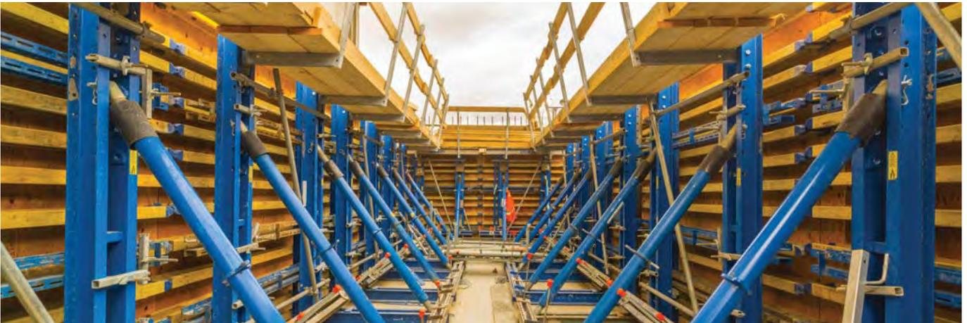
▲ Spillway Piers - Bullnose Custom Formwork
