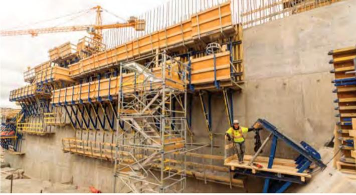
▲ Stair towers permit safe access to work decks.
