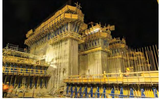
pressure for fast pouring rates. Since Framax is modular it was very flexible and fast to set up, requiring little skill. The strong steel frame of the Framax panel allowed an effortless stacking of panels to form tall walls with large openings. Staxo 100 Load-bearing system is used to support and pour the transfer slabs. Since crane access is limited in this area the towers can be dis-assembled manually and removed through a small opening. All components are lighter than 40 kg (88lbs.).
