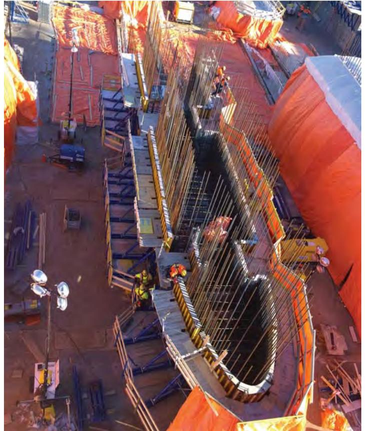
▲ D22 Dam formwork with large-area formwork Top 50
