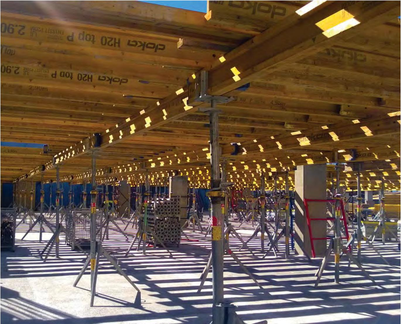
▲ Dokaflex is the fast, versatile floor-slab formwork for any desired layout. Any type of plywood can be used, so that any concrete surface finish can be achieved based on the requirement of the architect.
