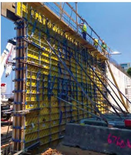
▲ The perfect panel size-grid gives you innumerable possible combinations, in both width and height. You can use the panels either vertical or horizontal, and the 6 in. increment grid allows for optimum adaptability of the formwork to the dimensions of the structure, at all times.
