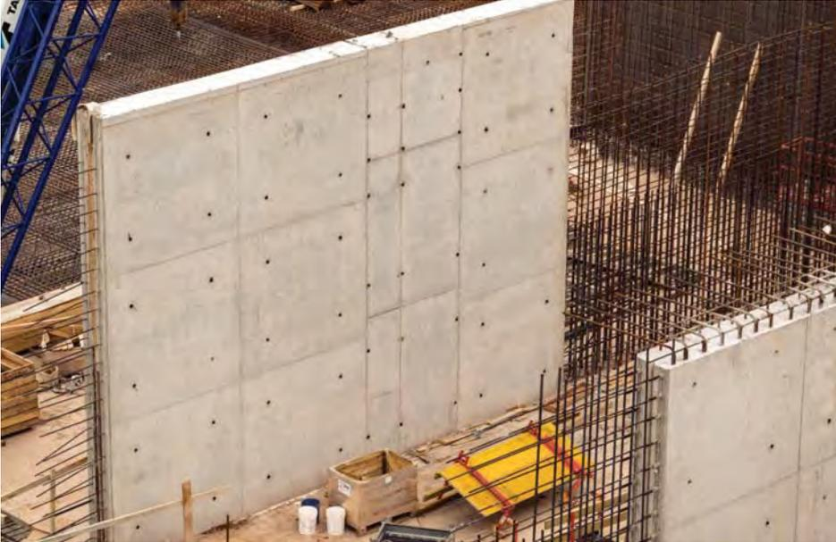
▲ Quality concrete finish was a requirement which Framax wall formwork was able to accomplish.
