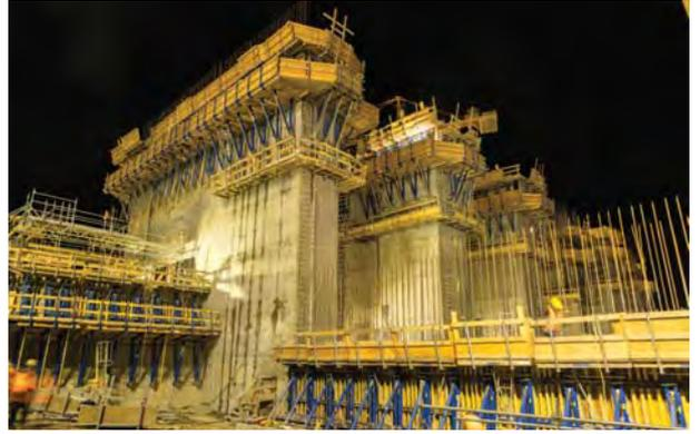
pressure for fast pouring rates. Since Framax is modular it was very flexible and fast to set up, requiring little skill. The strong steel frame of the Framax panel allowed an effortless stacking of panels to form tall walls with large openings. Staxo 100 Load-bearing system is used to support and pour the transfer slabs. Since crane access is limited in this area the towers can be dis-assembled manually and removed through a small opening. All components are lighter than 40 kg (88lbs.).
