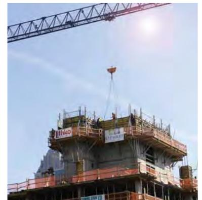
▲ Lithko used Frami universal column forms with its 1,650 psf pour pressures for the 50 ft tall columns and jumped them in multiple lifts.
