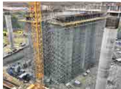
▼ 30,000 load-bearing tower frames complete the optimised solution.
