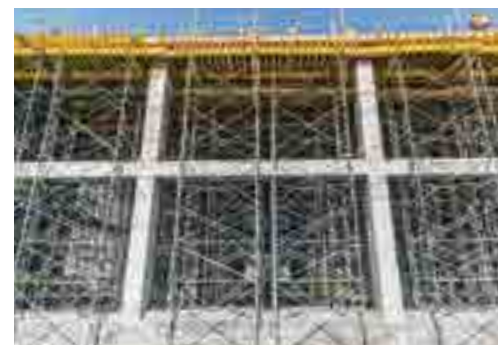
▲ Boosting productivity with the light weight shoring system Staxo 40.
