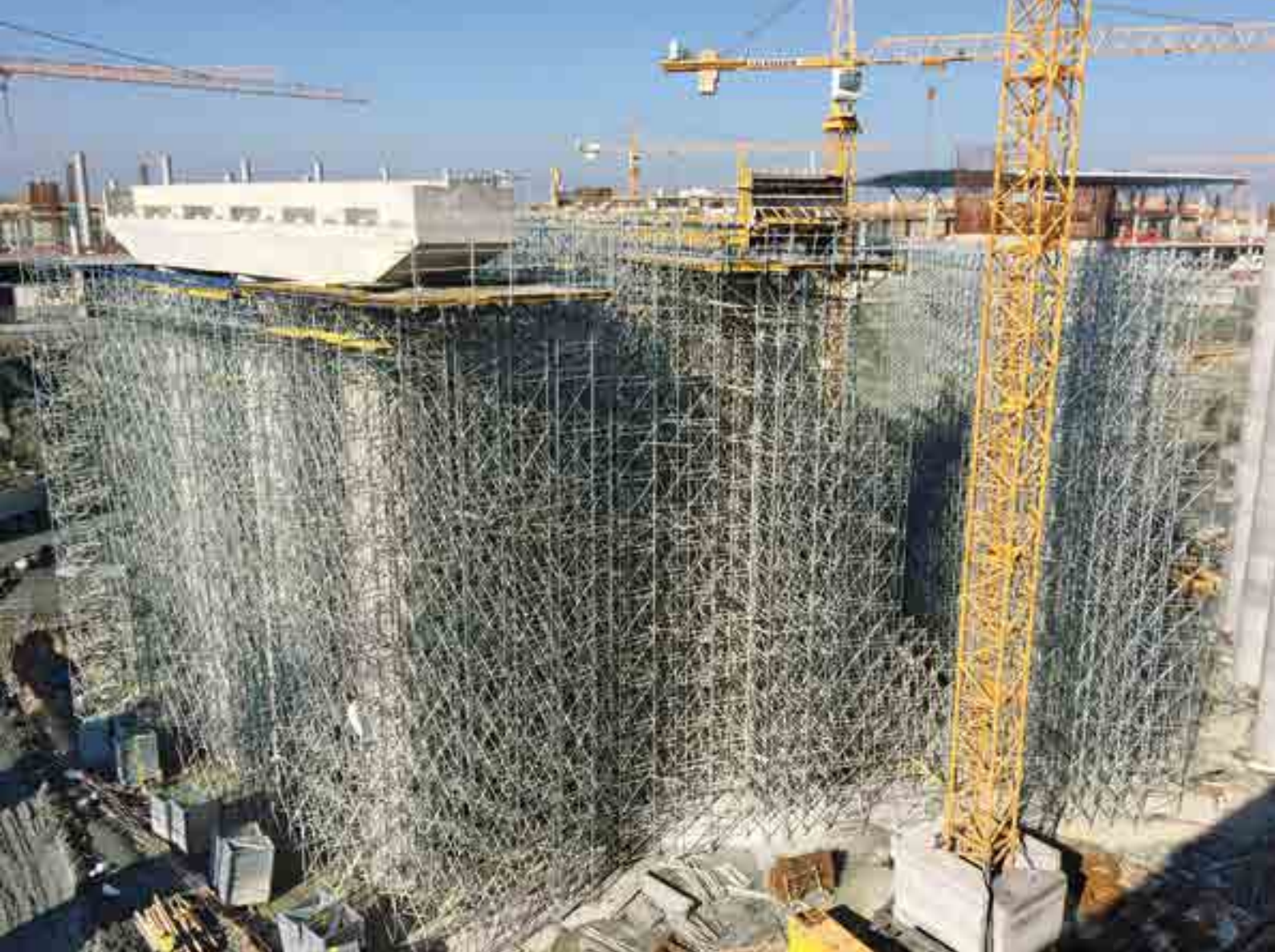
▲ Scaffolding for Istanbul's mega airport project.
