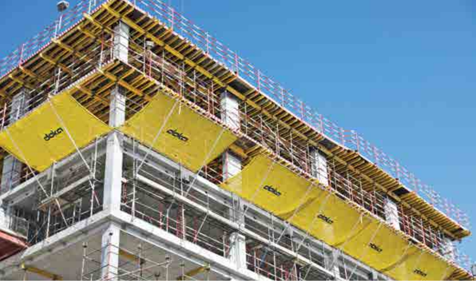
▲ Doka Safety Net Fan as part of the commitment to the wellbeing of site team members.
