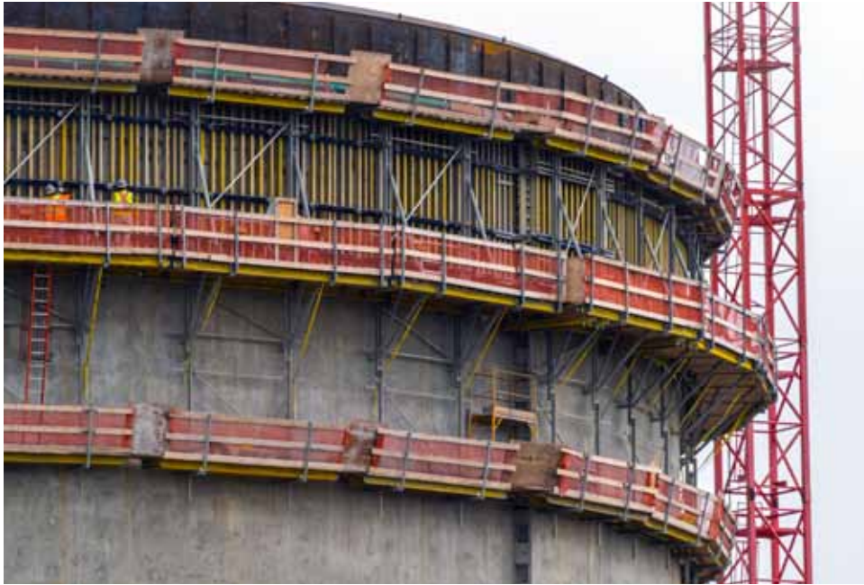
▲ The project is scheduled for completion in October 2016.
