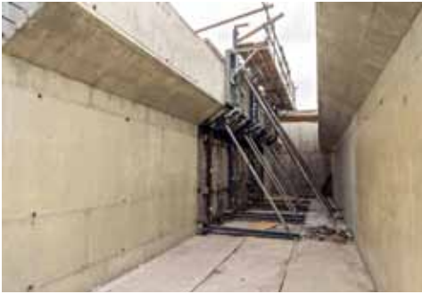
▲ Archer Western Contractors Ltd. is especially impressed with how fast crew members were able to cycle the Y wall forms.
