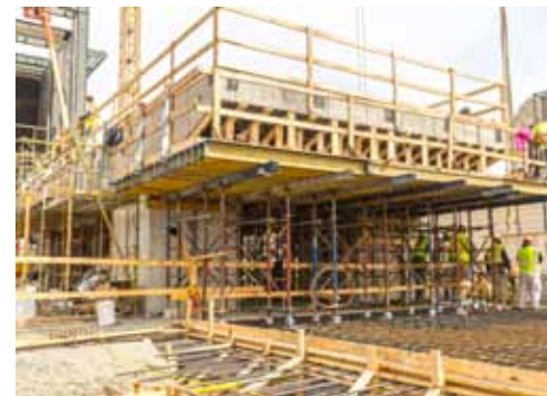
▲ Top slab supported with Doka's 10 Kip shoring
