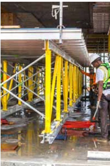
▲ The DokaTruss table represents the fastest method to set and strip large slab formwork.
