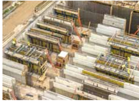
▲ Archer Western Contractors Ltd. is especially impressed with how fast crew members were able to cycle the Y wall forms.
