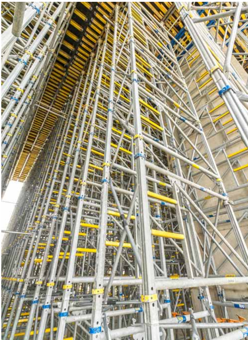
▲ Doka's Staxo 100 high capacity fast shoring system.
