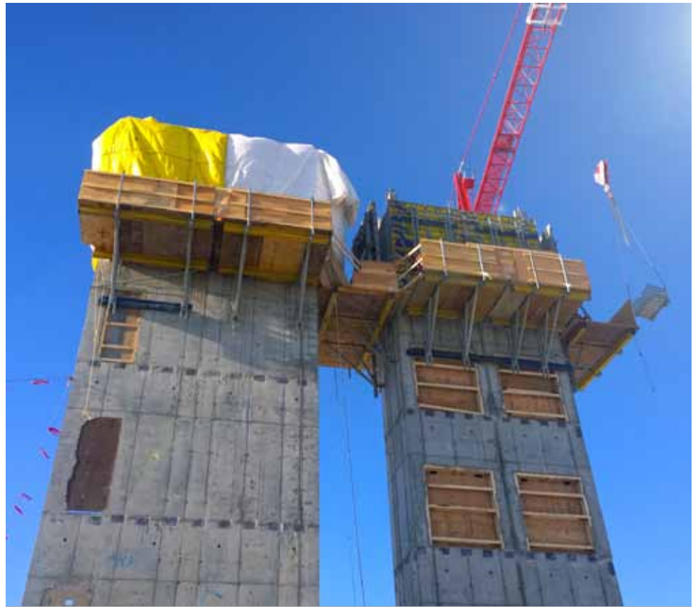
▲ Connected platforms allow for a safe work environment on both towers.
