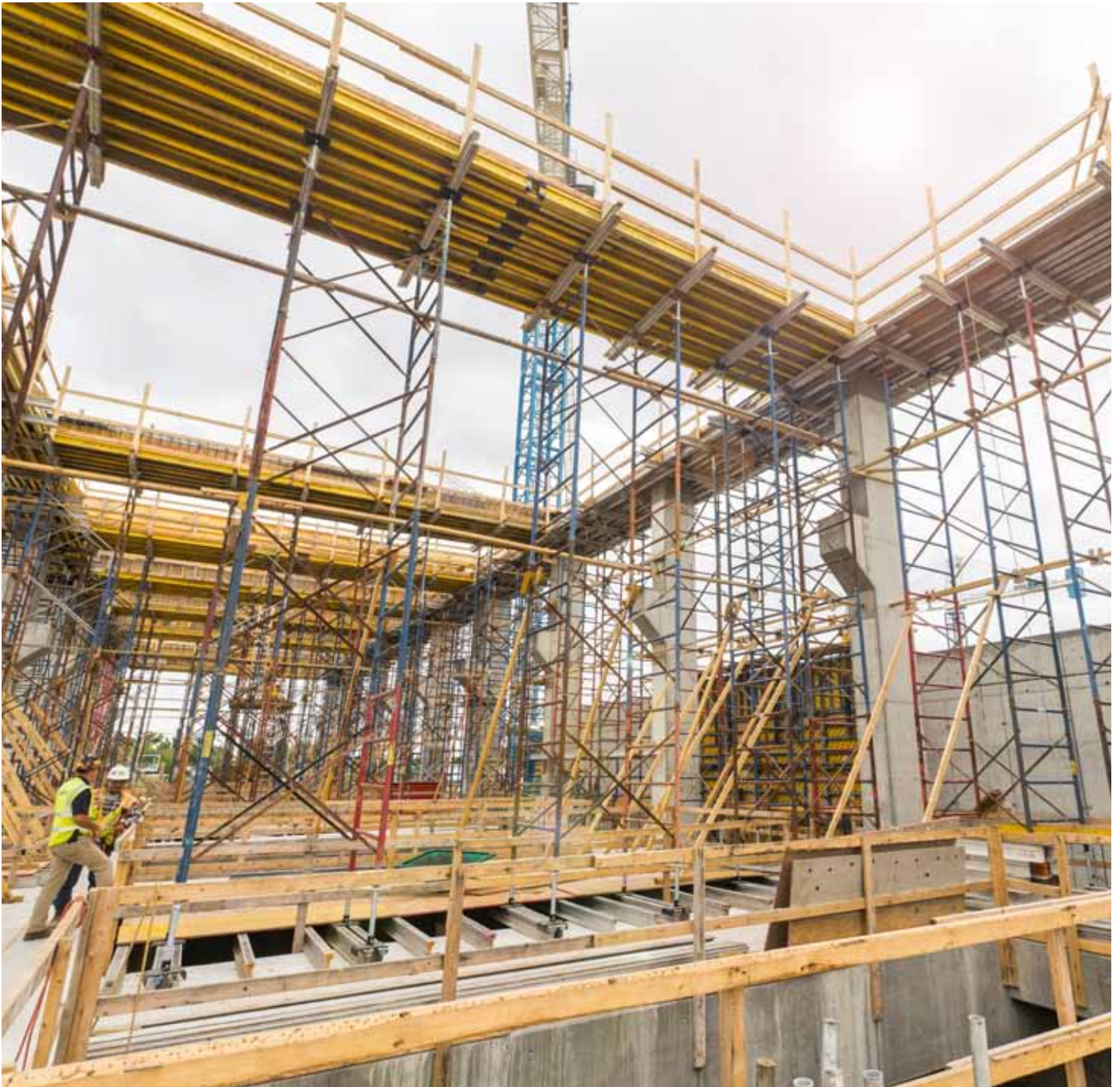
▲ Doka's 10 kip shoring was used for the high slabs and beams.
