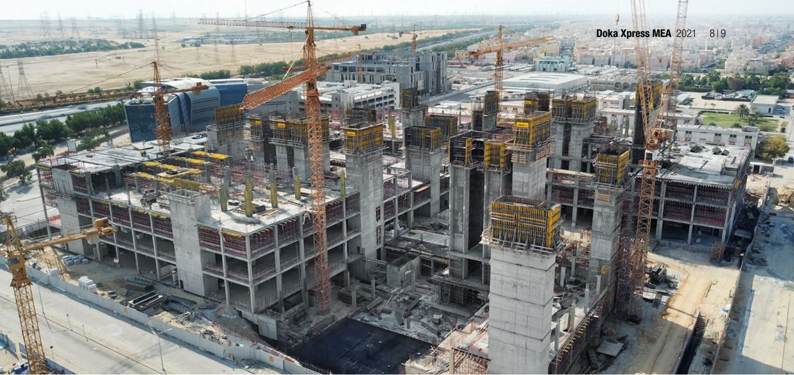
Climbing formwork 150F and Top 50 played an important role in the timely delivery of Al Adan.
