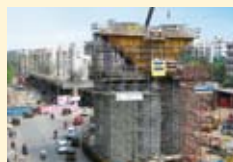
Mumbai metro rail bridge
