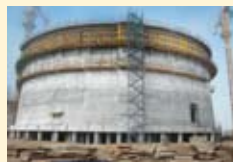
Double-walled storage tank, Dahej
