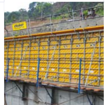
▲ Same set of formwork can be used for retaining walls of different sizes.
