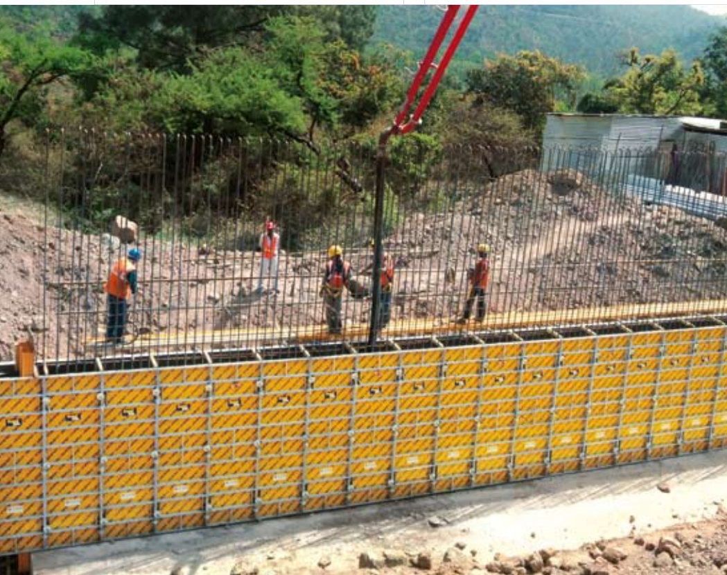
▲ Same set of formwork can be used for retaining walls of different sizes.
