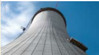
▲ Cooling tower formwork SK175 is a fully mechanized, self climbing large area formwork system.
