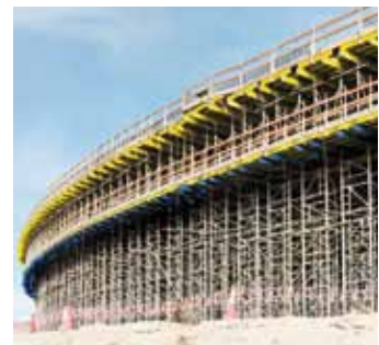
▲ Flexible standard systems such as Staxo 100 and Staxo 40, Doka slab formwork offers interesting system expansions for any shoring tower design.
