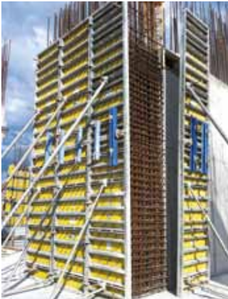
▲ Walls and columns are poured using Framed formwork Framax Xlife.
