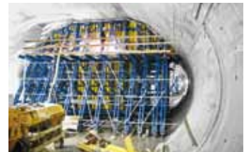
▲ Cross-section changes and varying structural geometries can be realised safely using the flexible Load-bearing tower SL-1.
