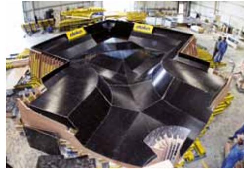
▲ The bridge deck formwork was assembled in advance.
