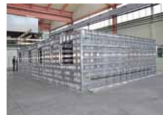
▲ With Doka OneGo walls and slabs are poured in one step.
