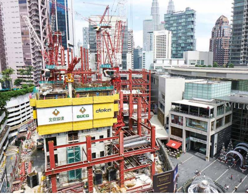
▲ Up to four climbing units are automatically climbed up to the next pouring section using innovative, double-acting mobile hydraulic cylinders. The hydraulic cylinders are operated easily and quickly by remote control.
