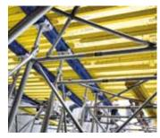
▲ The combination of hot-dip galvanised frames and diagonal crosses of d3 enables the towers to transmit loads up to 94 kN per leg.
