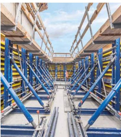
▲ The Dam formwork D22 with the integrated Platform system Xsafe plus is in use for the outer slope of the spillway.
