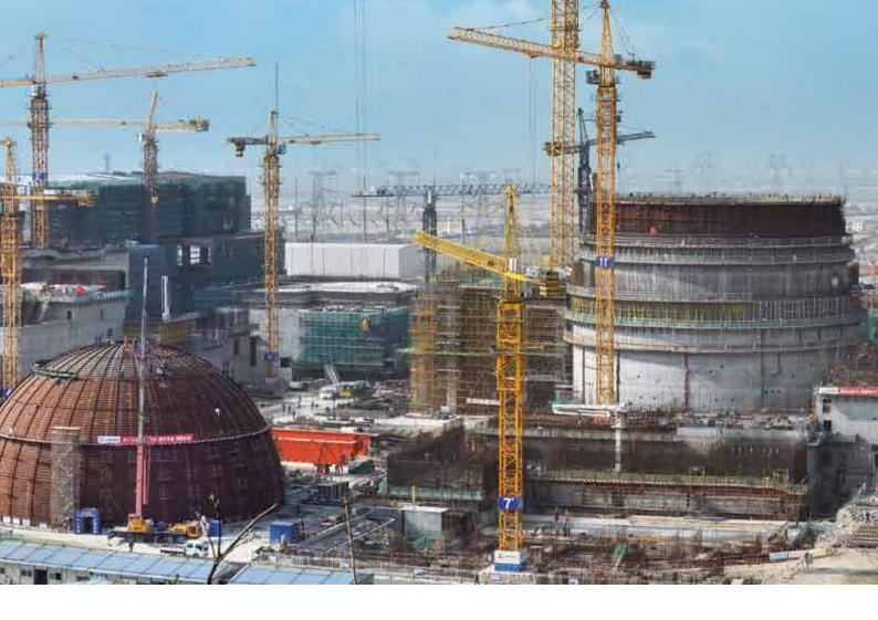
For the construction of double containment, one of the biggest challenges is the design of the formwork system. The gap between the inner and outer shells is only 1.8 m, so careful consideration must be given to the available space — especially in terms of whether or not the formwork hoisting and retracting distance can be guaranteed, and if there is sufficient operating space.
