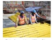
▲ Timber formwork beam H20 eco P is easy to handle and weighs only 5.2 kg.
