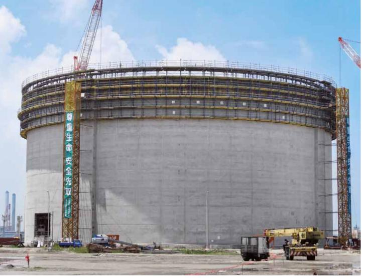
▲ The LNG tanks are erected with Large-area formwork Top 50 and Climbing platform D15.
