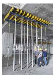
▲ Dokamatic tables are ideal for fast forming of large floor areas. At Singtel Data Centre West, they are used for forming slabs of 30 cm up to 1 m in thickness.
