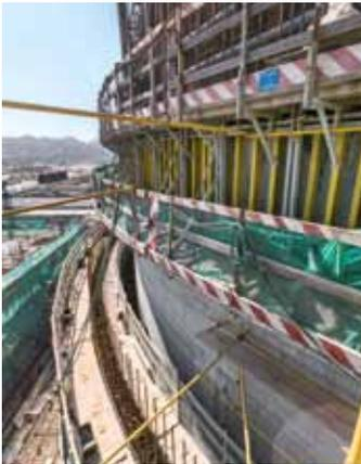
▲ The spacing between inner shell and outer shell is only 1.8 m, posing a challenge for the design of the formwork system.
