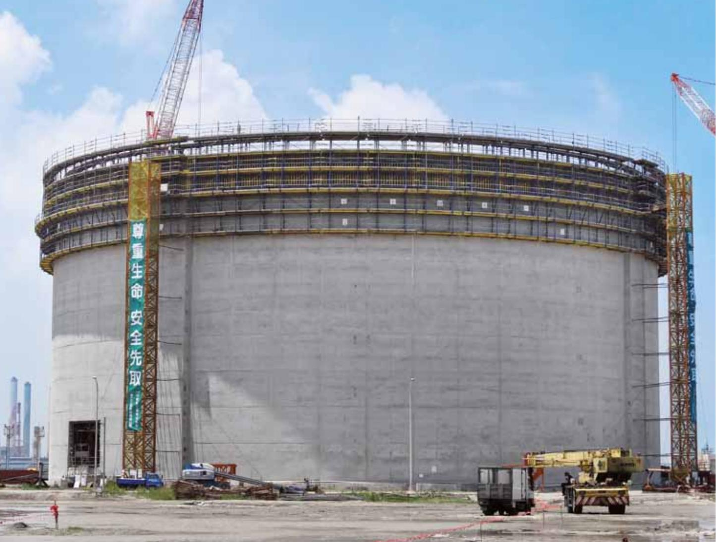
▲ The LNG tanks are erected with Large-area formwork Top 50 and Climbing platform D15.
