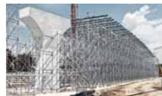
▲ The Load-bearing tower d3 scores with high load capacity, fast assembly and a broad spectrum of application.
