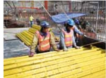
▲ Timber formwork beam H20 eco P is easy to handle and weighs only 5.2 kg.
