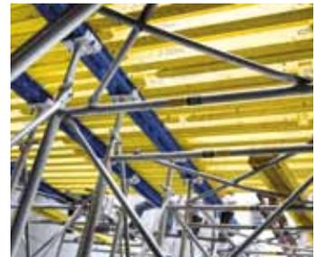
▲ The combination of hot-dip galvanised frames and diagonal crosses of d3 enables the towers to transmit loads up to 94 kN per leg.
