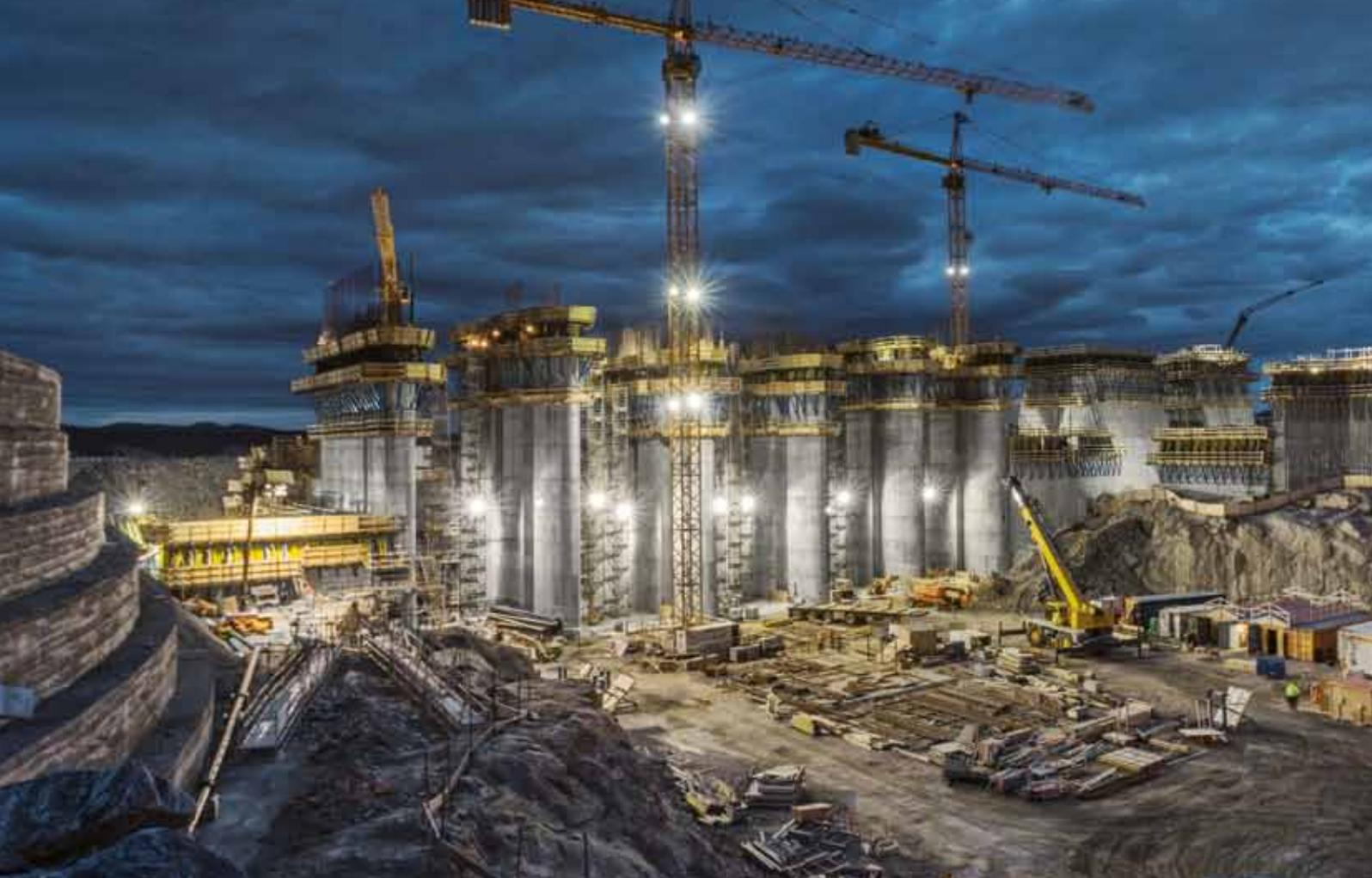
▲ Downstream view from right to left: North Transition Dam, 6 Spillway Piers, Centre Transition Dam, Separation Wall
