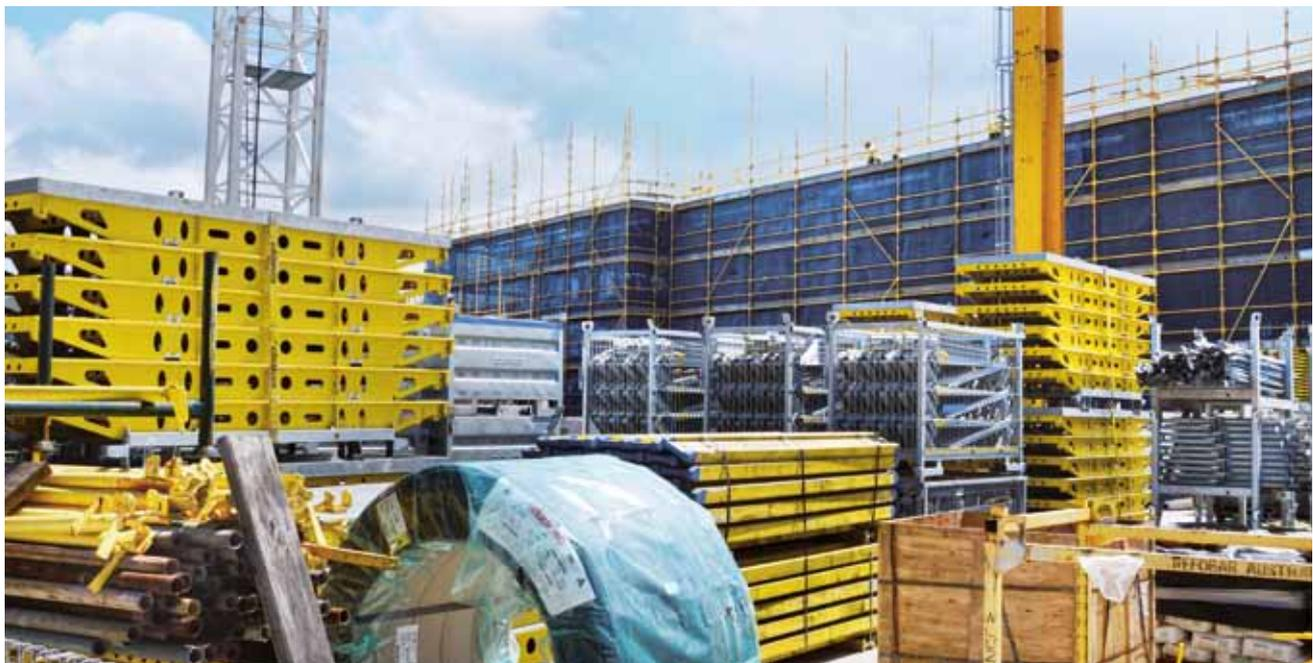
For Xayaburi Hydroelectric Power Project, Doka supplies 36,000 frames of Load-bearing tower d3, which is designed specifically for large shoring heights and high loads.
