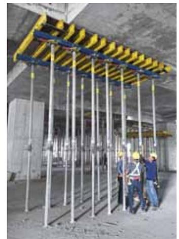
▲ Dokamatic tables are ideal for fast forming of large floor areas. At Singtel Data Centre West, they are used for forming slabs of 30 cm up to 1 m in thickness.
