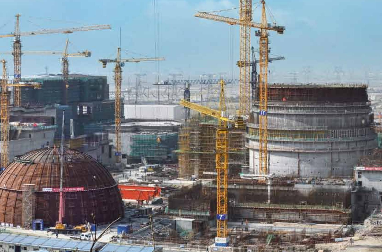
For the construction of double containment, one of the biggest challenges is the design of the formwork system. The gap between the inner and outer shells is only 1.8 m, so careful consideration must be given to the available space – especially in terms of whether or not the formwork hoisting and retracting distance can be guaranteed, and if there is sufficient operating space.
