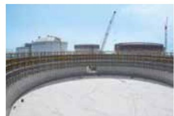
▲ The inner diameters of the tanks are 78 m.
