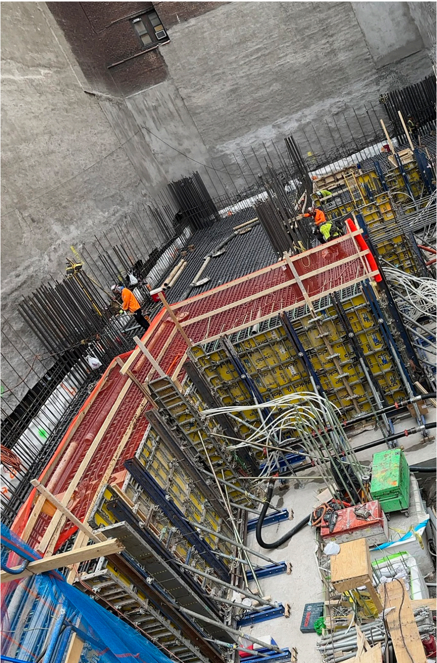
Cut Conditions Frami was the perfect system to adapt to cut-up geometry of the interior foundation walls.
