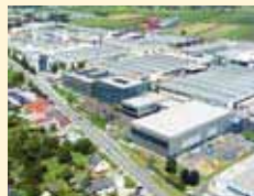
Doka's central plant
