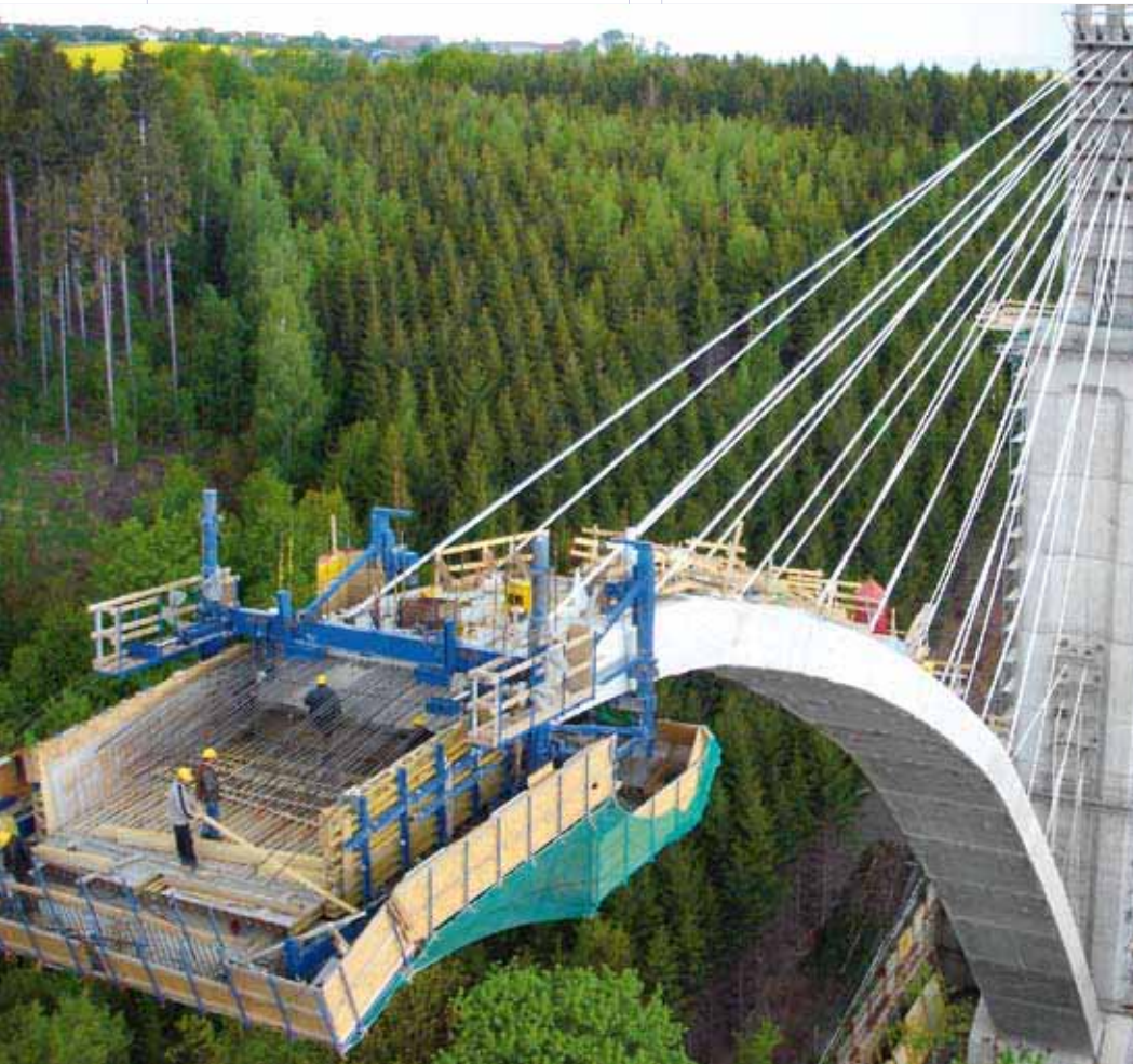
◀ The Seidewitztal Bridge in Germany was built with the Doka forming traveller.
