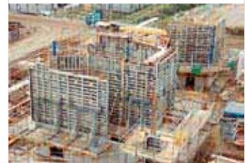
First building site with Framax framed formwork.
