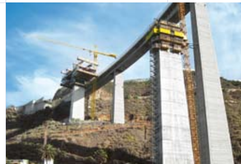
▲ The main piers of Viaducto 5 are being built with Doka’s automatic climbing formwork SKE 50 and Large-area formwork Top 50 in a four-day cycle.
