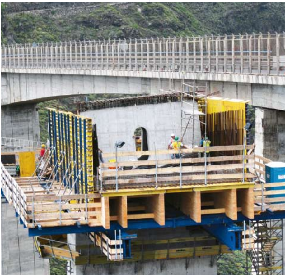
▲ The main piers of Viaducto 5 are being built with Doka’s automatic climbing formwork SKE 50 and Large-area formwork Top 50 in a four-day cycle.
