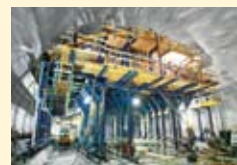
Gotthard Base Tunnel
