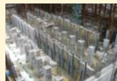
Kanamachi water treatment plant
